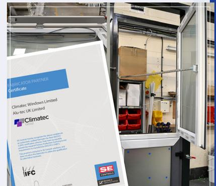
Automatic Opening Vents (AOVs) or smoke ventilation systems are designed to help ventilate and extract smoke from buildings during emergencies and in the event of a fire to facilitate the safe escape of occupants. Customers
